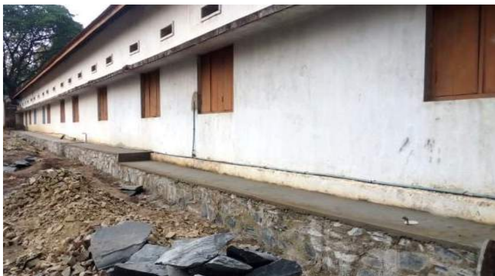
Renovated foundation work of the Building
